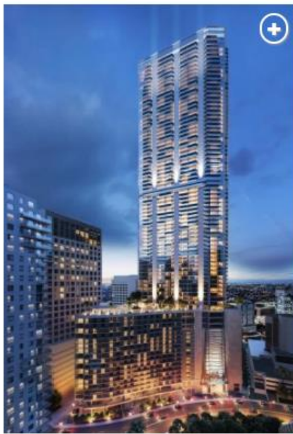
The Panorama Tower — Florida’s tallest building — will be the pinnacle of ultra luxury when it opens next year.
