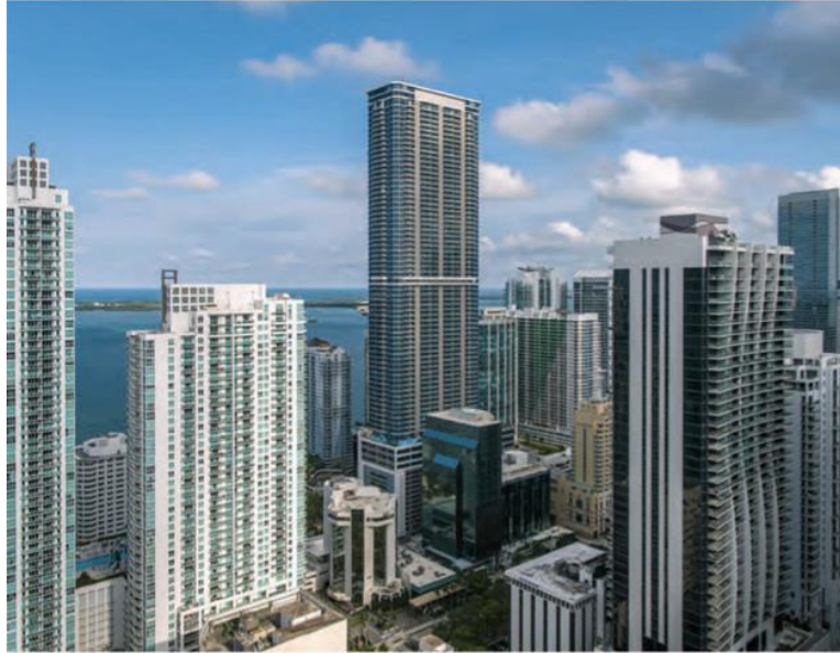
The 85-story Panorama Tower is the tallest residential building on the East Coast, south of New York City.
