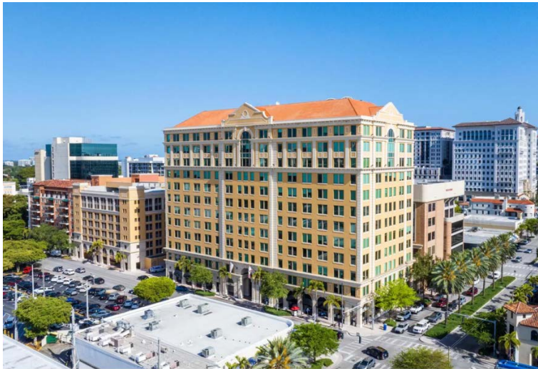
Courtesy of Intalex, Itero and Greenwall Capital Management The Ponce at 2525 Ponce de Leon in Coral Gables
