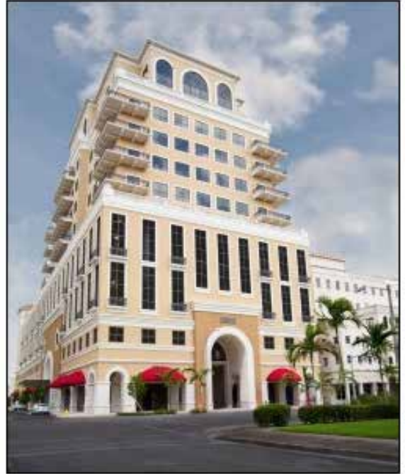
The office and retail building at 2020 Ponce De Leon Boulevard
